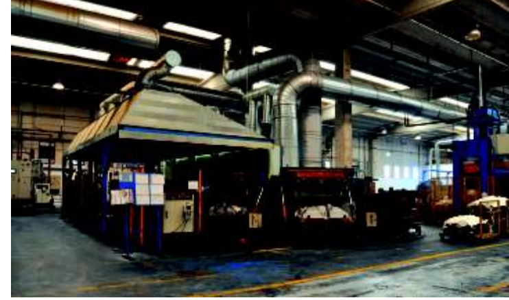
A view of Adler's spray and foaming plant for FIAT's dash insulators near Matera, Italy.
